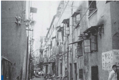
picture 'Comfort Station' in Wuhan, China
